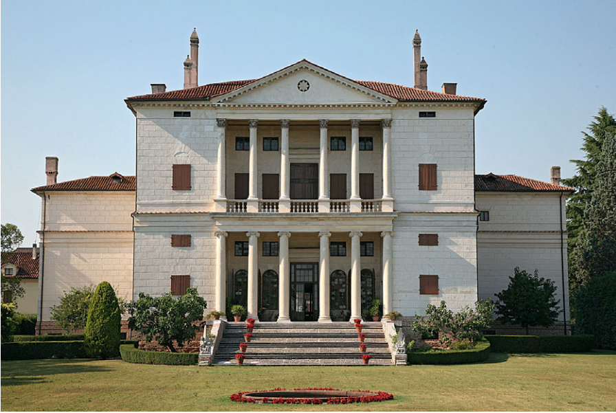
19. Andrea Palladio, Villa Cornaro, Piombino Dese, south facade, 1552–54. Photo: Wikimedia Commons, Hans A. Rosbach, CC BY-SA 3.0
