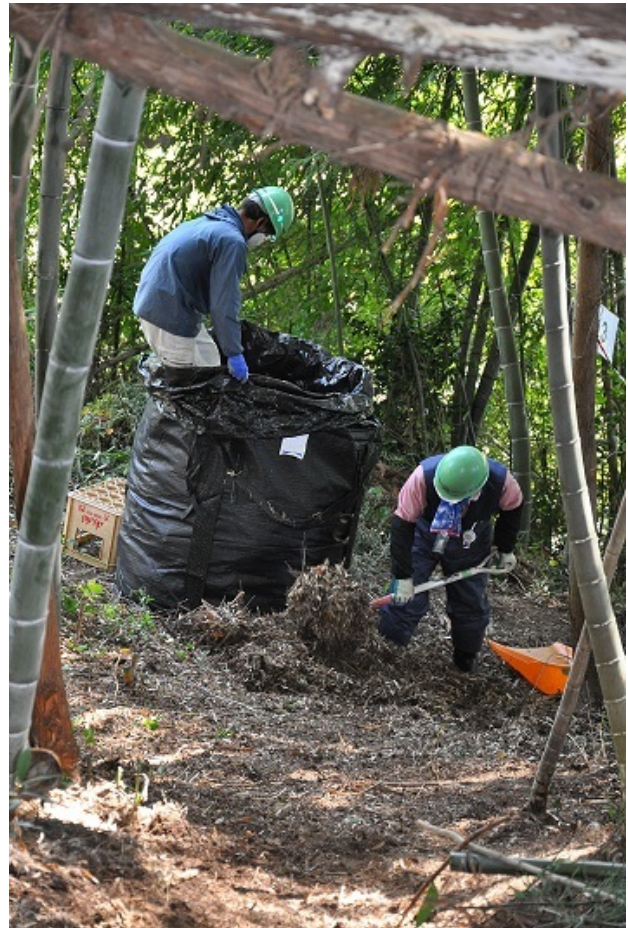
Decontamination work, Nihonmatsu, Fukushima. Image credit: Peter Wynn Kirby.
